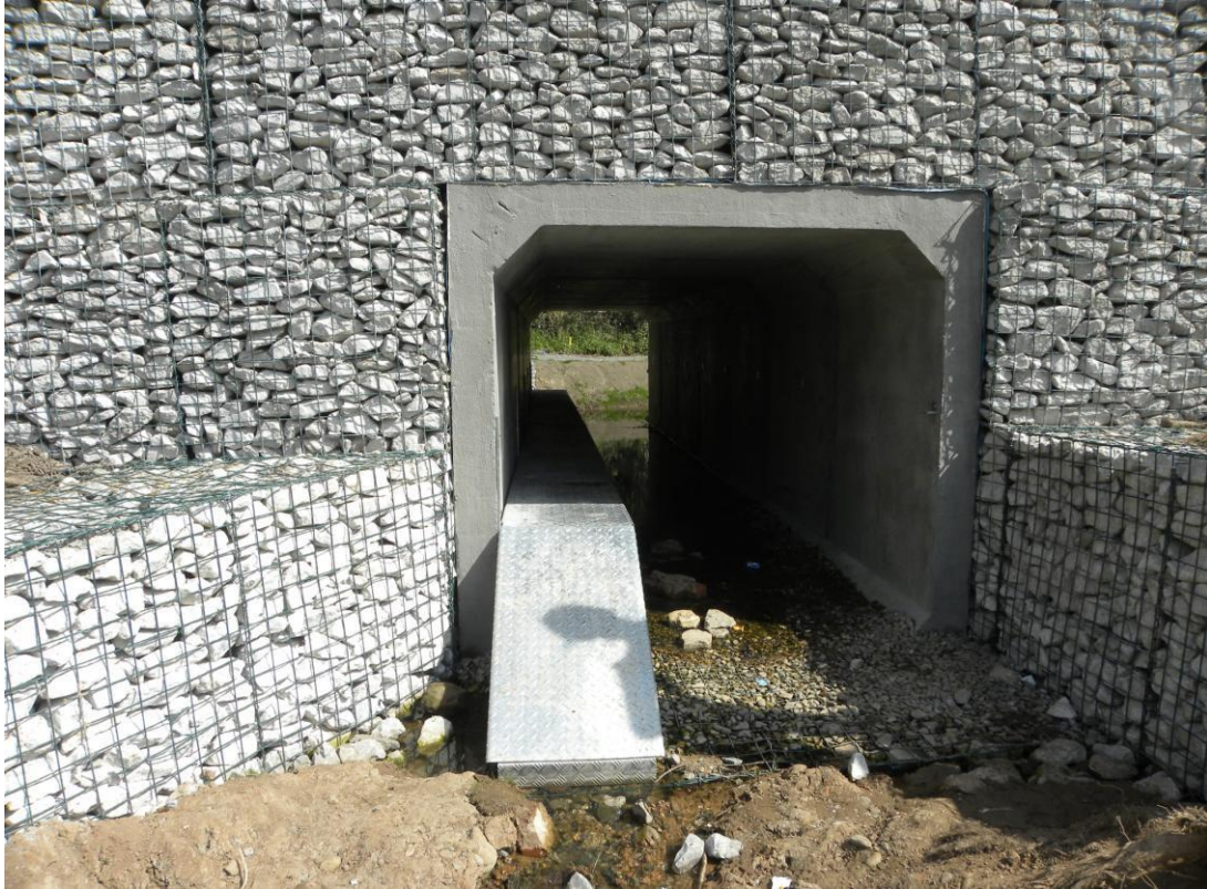
Otter ledge incorporated into a road culvert as a feature to allow the upstream movement of otters at times of spate conditions (Photo R. Parry)
