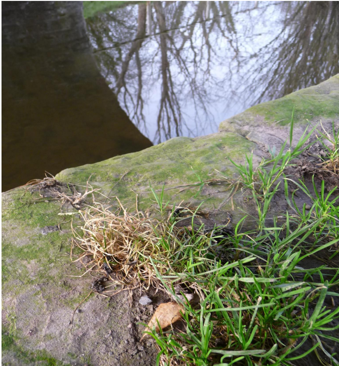
Otter spraints of various ages on masonry under a bridge over the Brecon and Monmouth Canal within the Usk catchment. Acids leaching from the spraints have turned the grass brown. (Photo: R.Strachan)
