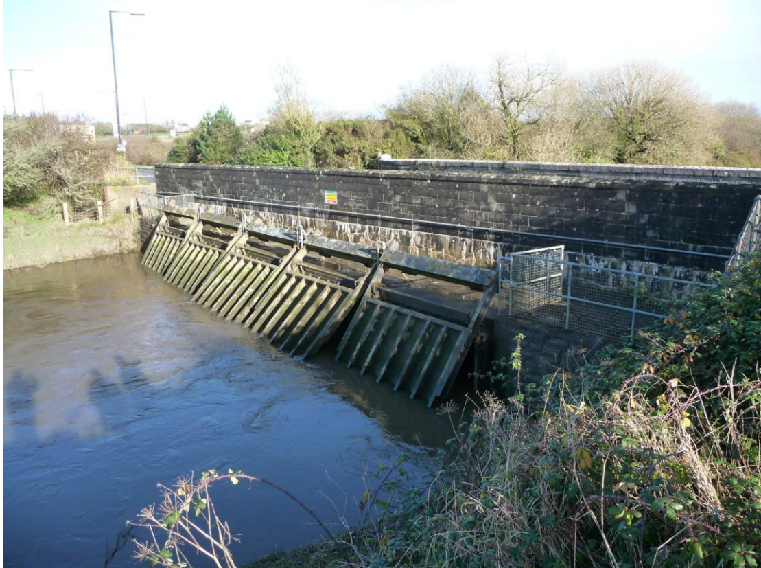
Tidal flaps on the Gwendraeth Fawr may be a barrier to otters travelling the estuary that will force them to cross the busy A484 near Kidwelly (Photo: R. Strachan)
