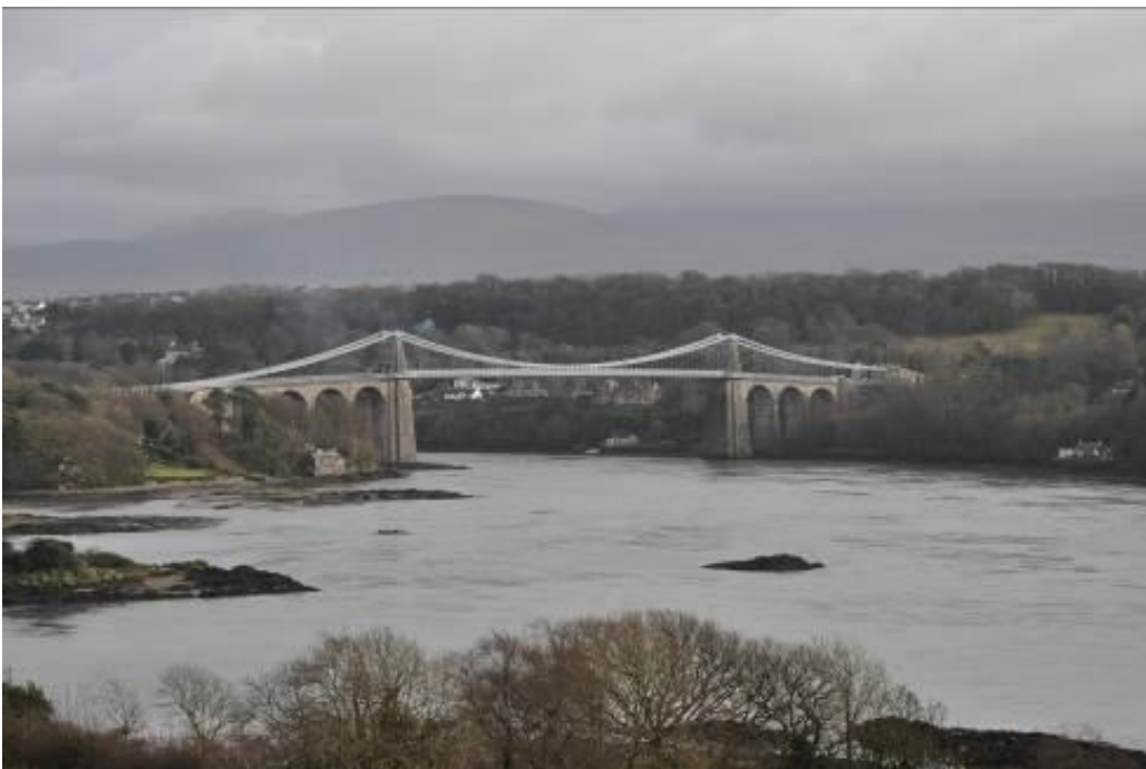
Menai Suspension Bridge
