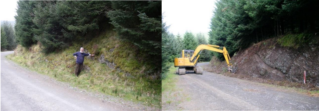
Figure 21 Geological SSSI before site clearance before (left) and after (right)
