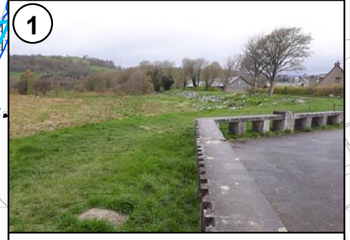
1 LAKE EMBANKMENT LOOKING WEST ACROSS THE PROTECTED SITE, FROM THE 'BANDSTAND' SEATING AREA
