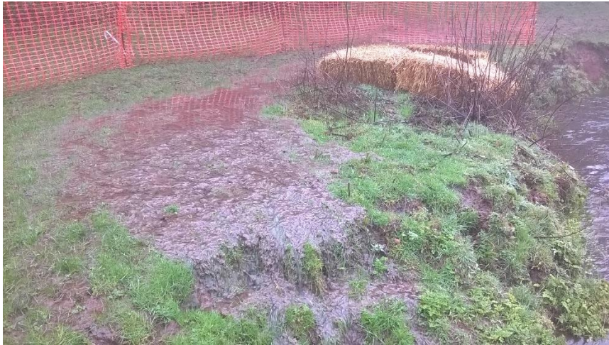
Figure 30 A surcharging sewer causing pollution of a river (Source: NRW).
