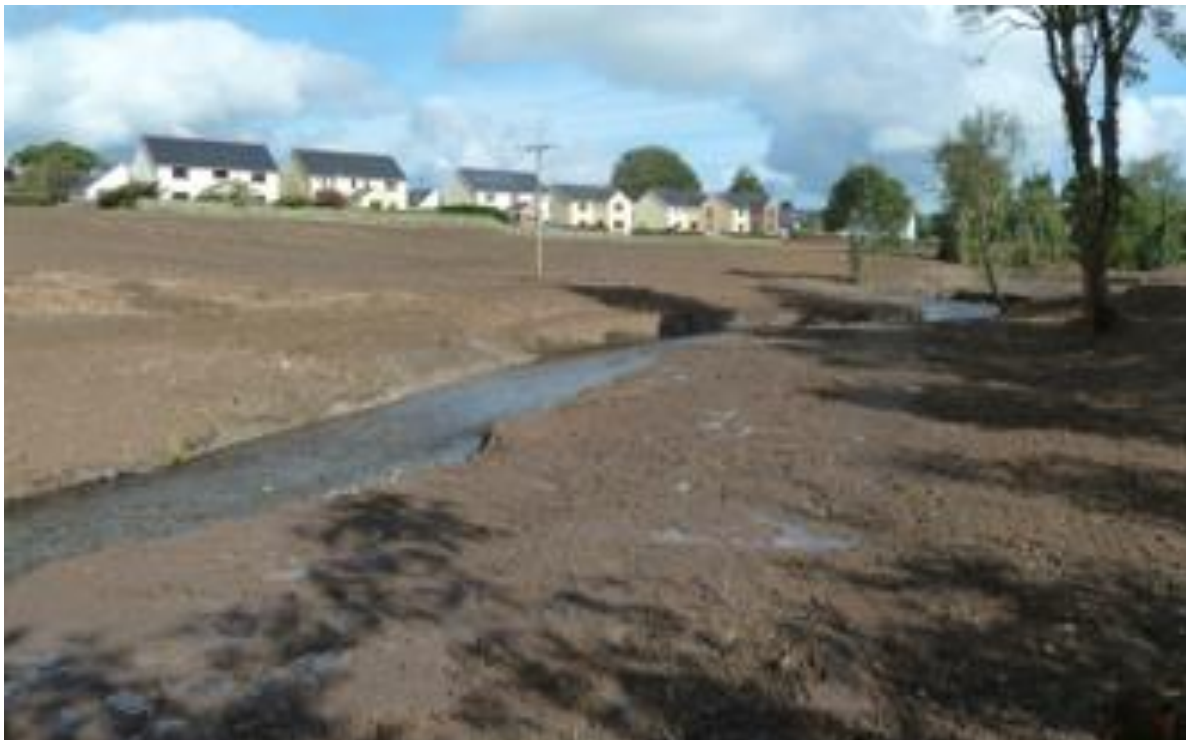
Figure 18 River straightening, soil erosion and destruction of river corridor habitat (this section has since been colonised by invasive non-native plants). This is an example of unconsented river modifications (the example shown has occurred since 2017) ) (Source: NRW).
