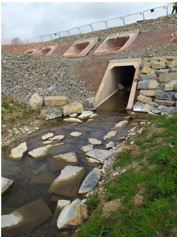
Figure 21 Culvert installed as part of road scheme- 2017-2019 (Source: NRW).
