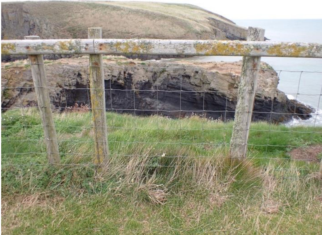
Figure 40. Example of the fence around Carreg Lydan (Location A).
