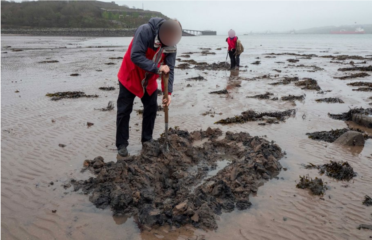
Figure 93 - Control hole 1 being dug with control hole 2 in background, 28/11/2019.
