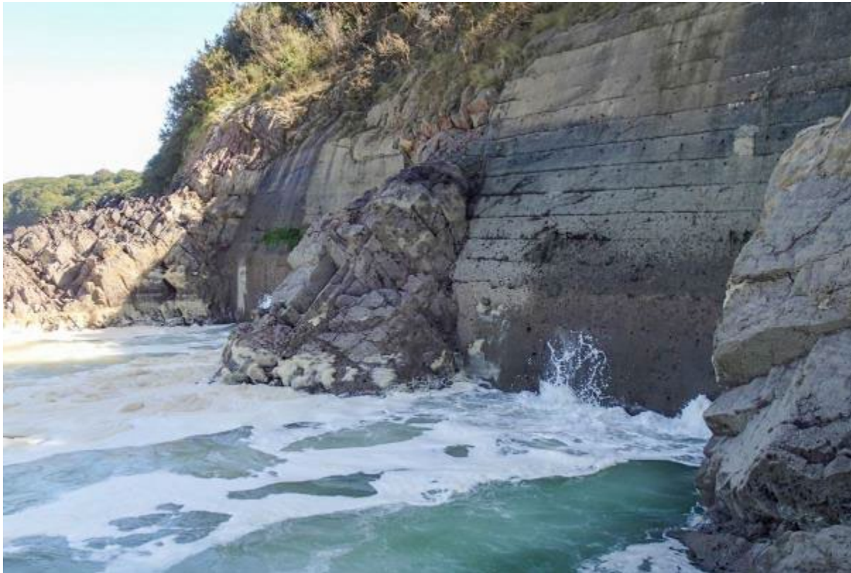
Figure 81. Foaming waste-water exiting the Pembroke Power Station cooling water outfall. (Date of photo 5 th September 2012)
