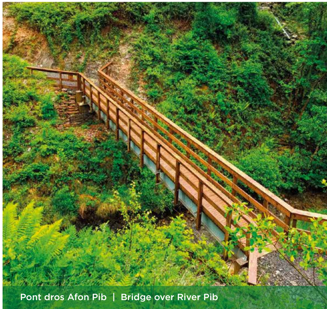
Pont dros Afon Pib | Bridge over River Pib
