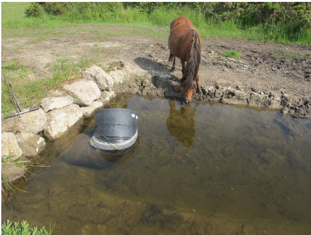
Adjustable pipe intake in a pool with stock-friendly margins. Adjustment of the pipe elbow can raise or lower levels by c. 0.7 m. This pipe serves to enable drainage freeboard from 3 rd party land to the right whilst allowing rewetting of fen to the left. Photo: P.S. Jones/Anglesey & Llyn Fens LIFE Project.
