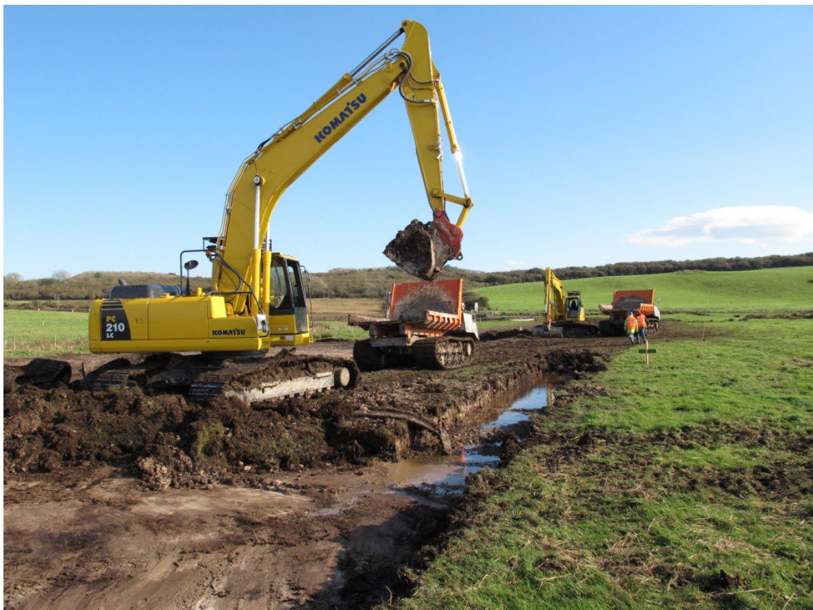
Turf and peat stripping at Cae Gwyn, Cors Erddreioniog, Anglesey. Photo: P.S. Jones/Anglesey & Llŷn Fens LIFE Project.
