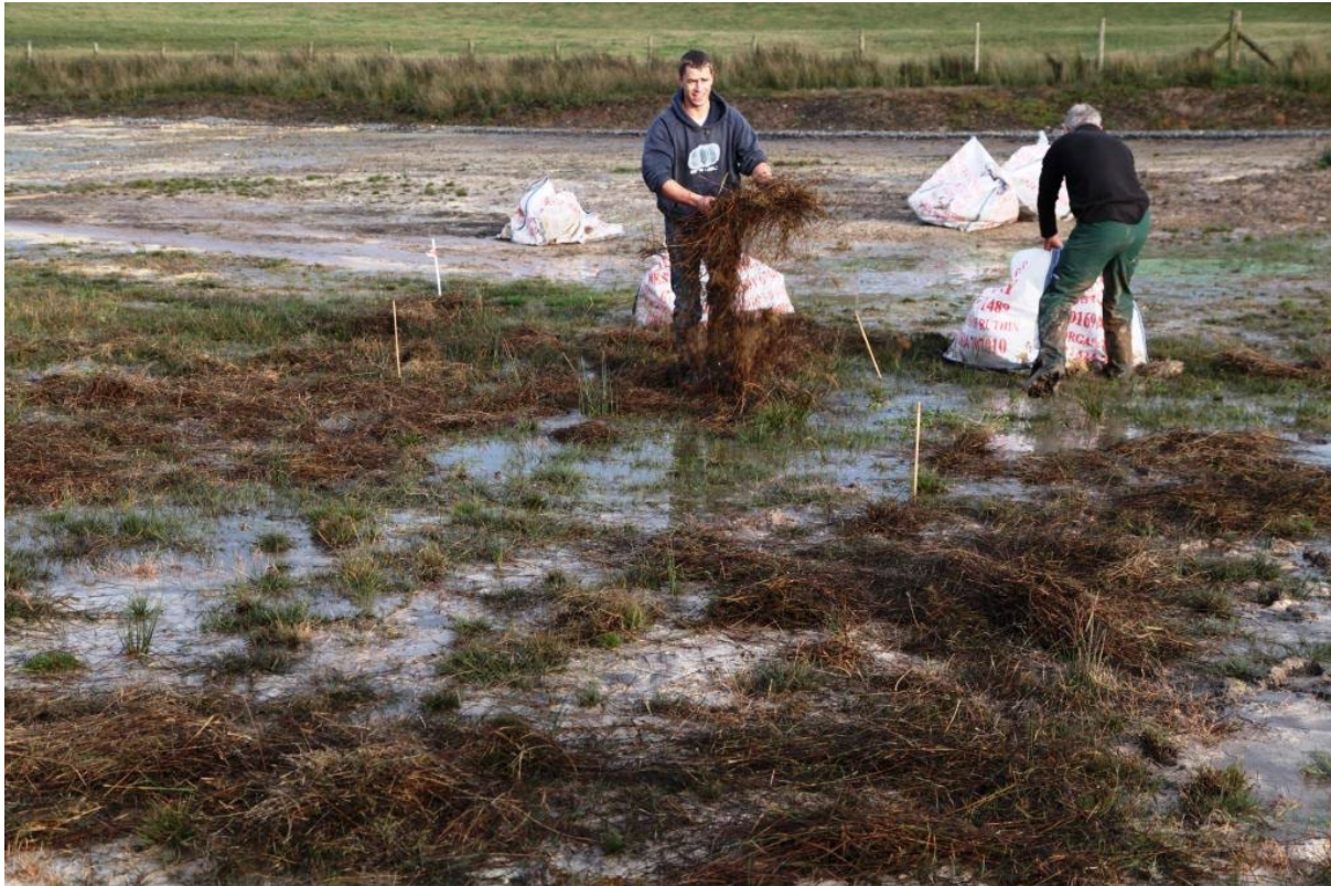
Llion Jones and Emyr Humphreys of NRW spreading green hay onto the artificially stripped wet peat and marl surface at Cae Gwyn, Cors Erddreiniog, Anglesey. Photo: P.S. Jones/Anglesey & Llyn Fens LIFE Project.
