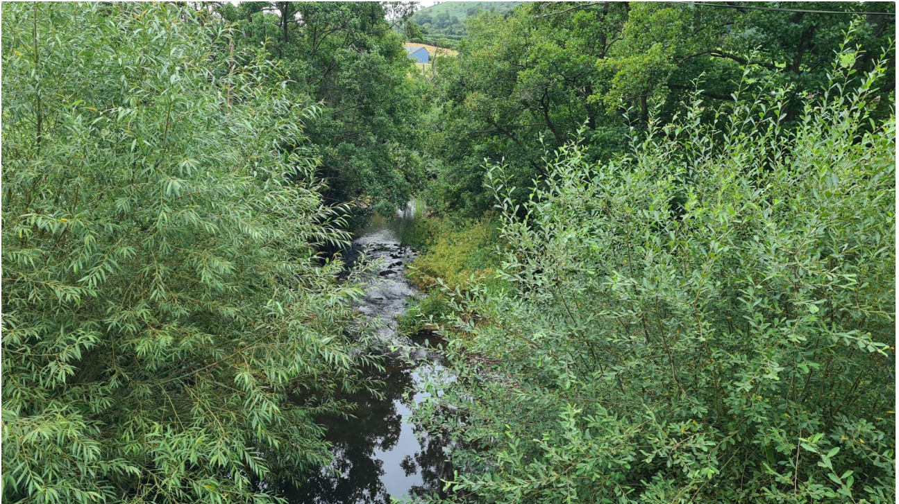
Figure 43. Photo of Edw, Cregrina, from the road bridge facing downstream
